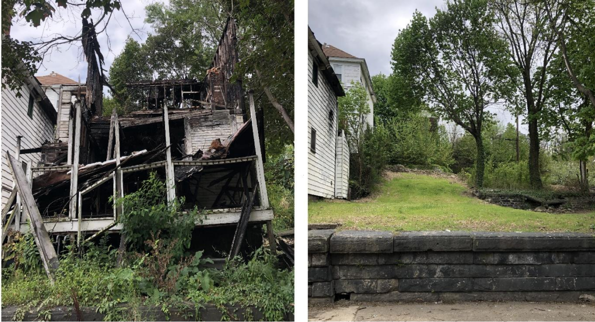
Figure 4 – Before & After Demolition at 512 College
