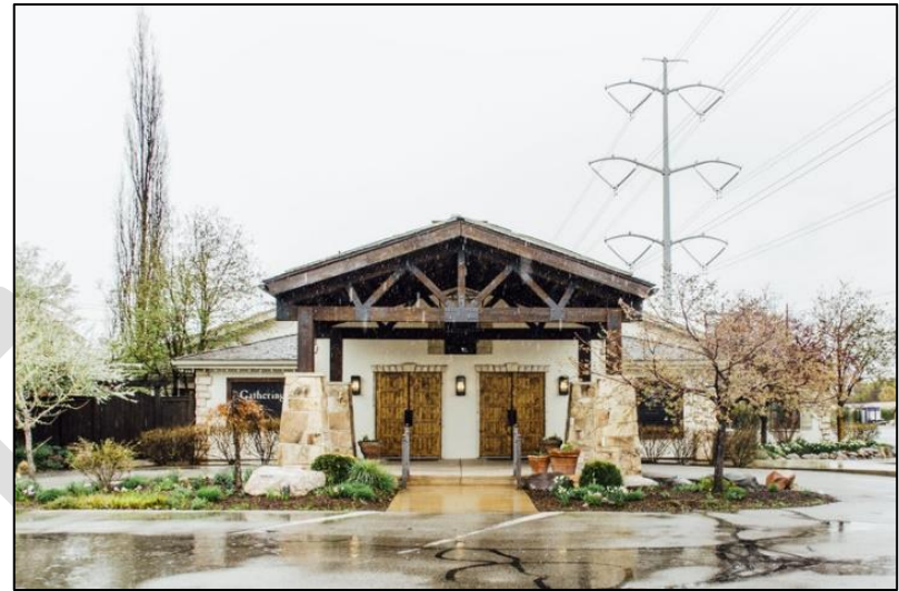
Figure 5—Gardner Village Conference Center
